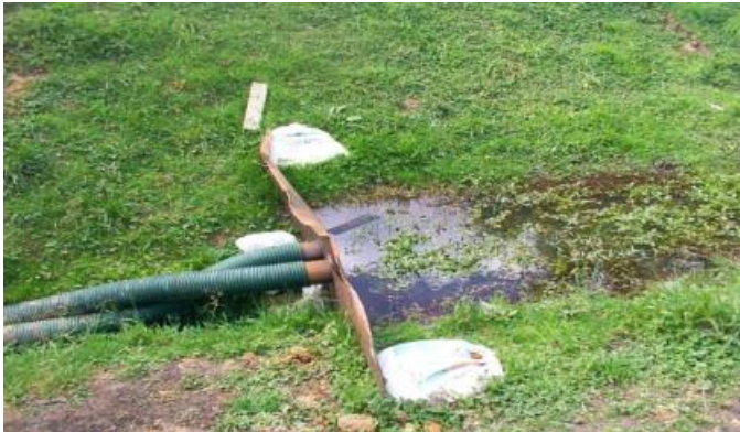
Figure 4 Example of dam and pumping diversion (New Zealand Transport Authority, 2014. Erosion and Sediment Control Guidelines for State Highway Infrastructure)
